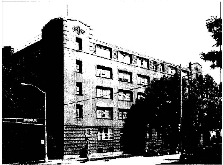
The Kleuter Wholesale Grocery Warehouse, more recently the Mautz Paint factory, at 901 E. Washington Ave., was designed in a Prairie-style by prominent Madison architect Alvan Small in 1915.
